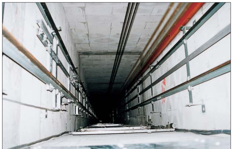
Blick in den Schacht (118 m) View into hoistway (118 m) Vue en gainé (118 m)
